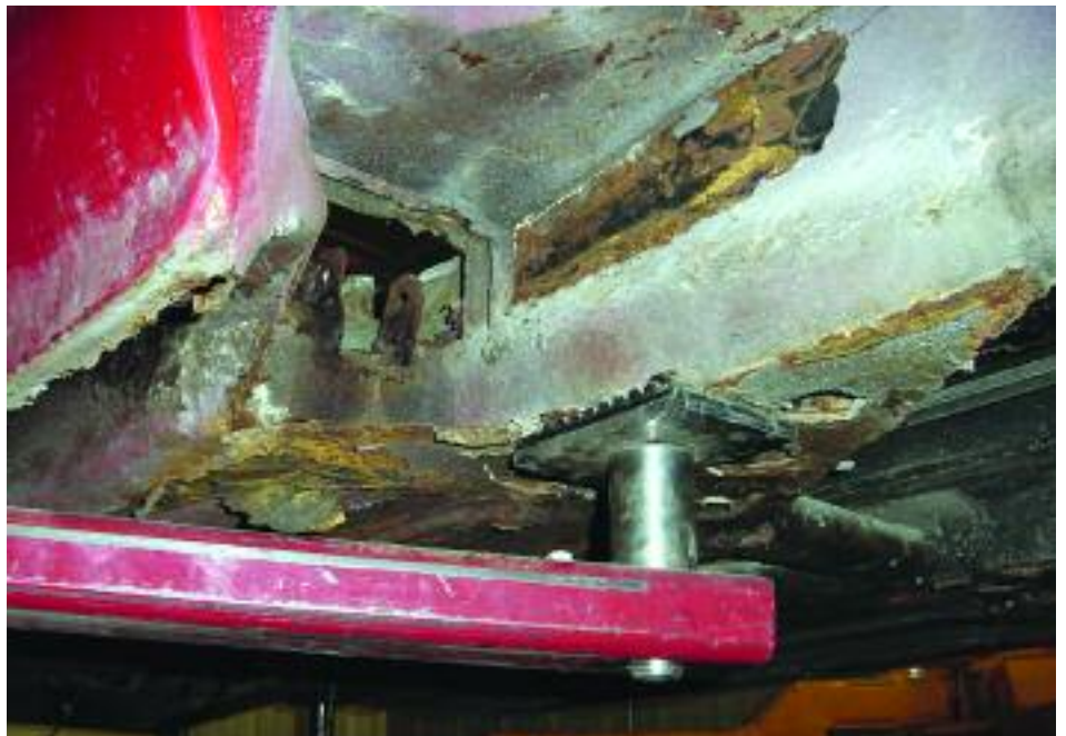
Rust in sill to floor area.
